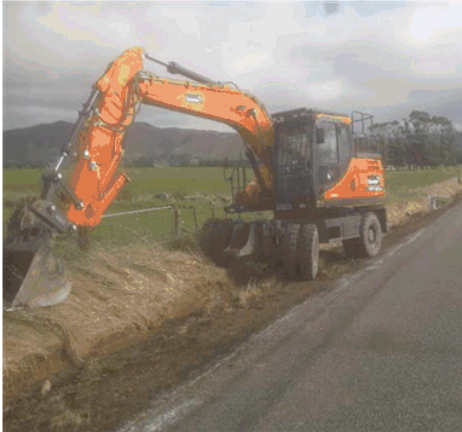
Our new wheeled excavator completing drainage work in preparation for our reseals
