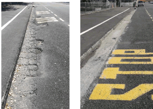
Sump repairs, before and after, Bridge St Eketahuna
