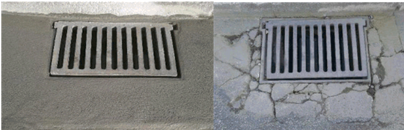
Before and after - Repairs to the bus stop outside St Josephs School, Mcphee St, Dannevirke
